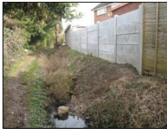
*A riparian ditch in need of maintenance to remove vegetation, silt and debris*
