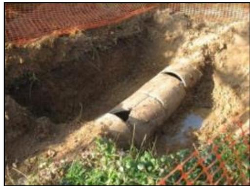
*A damaged culvert requiring repair*
